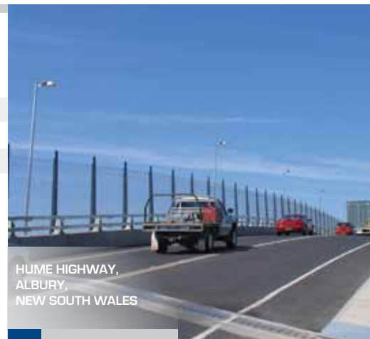
Urban 42W Lynx-CFTE H = 6.5m Upcast = 5 deg
