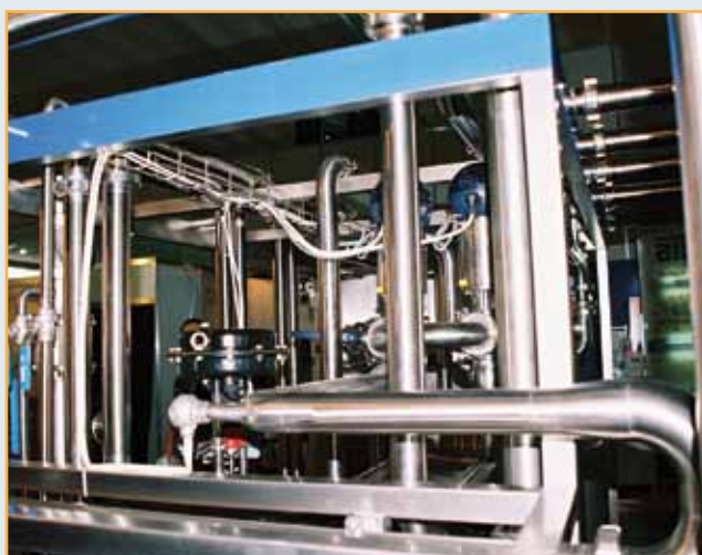
Welded onto machine frames
