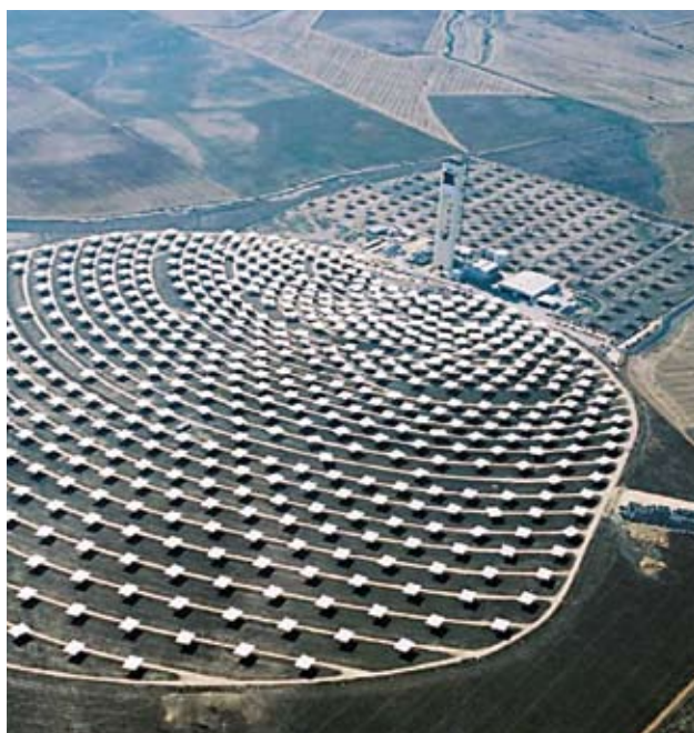
Figure B.8 – Central receiver plant
