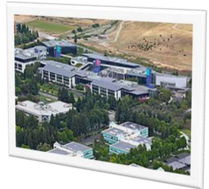
Rooftop photovoltaic power station at Googleplex, California
