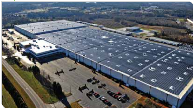
> 5.2 MW power plant (North Carolina, USA)
