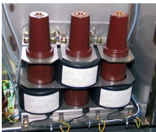
Bottom view of toroidal type current transformers on external-cone cable plug-in terminals (T2 Function)
