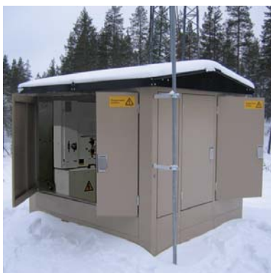
Compact substation
