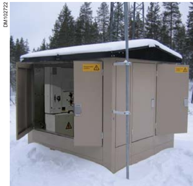
Compact substation
