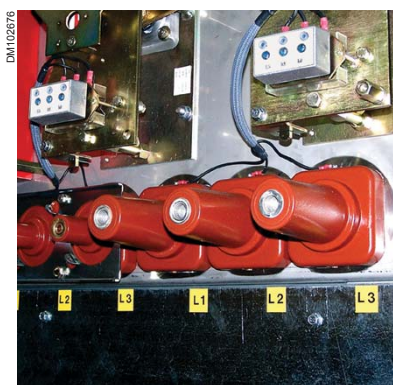
Cable connection bushings (page 14, item 9)
