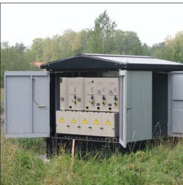
Compact substation
