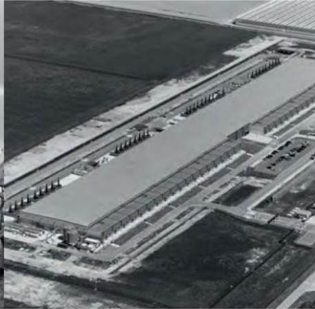
Google Data Center Netherlands
