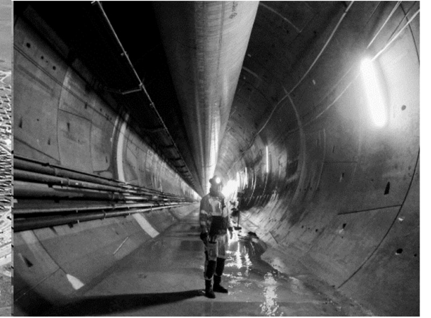
Follo Line Railway Tunnels Norway
