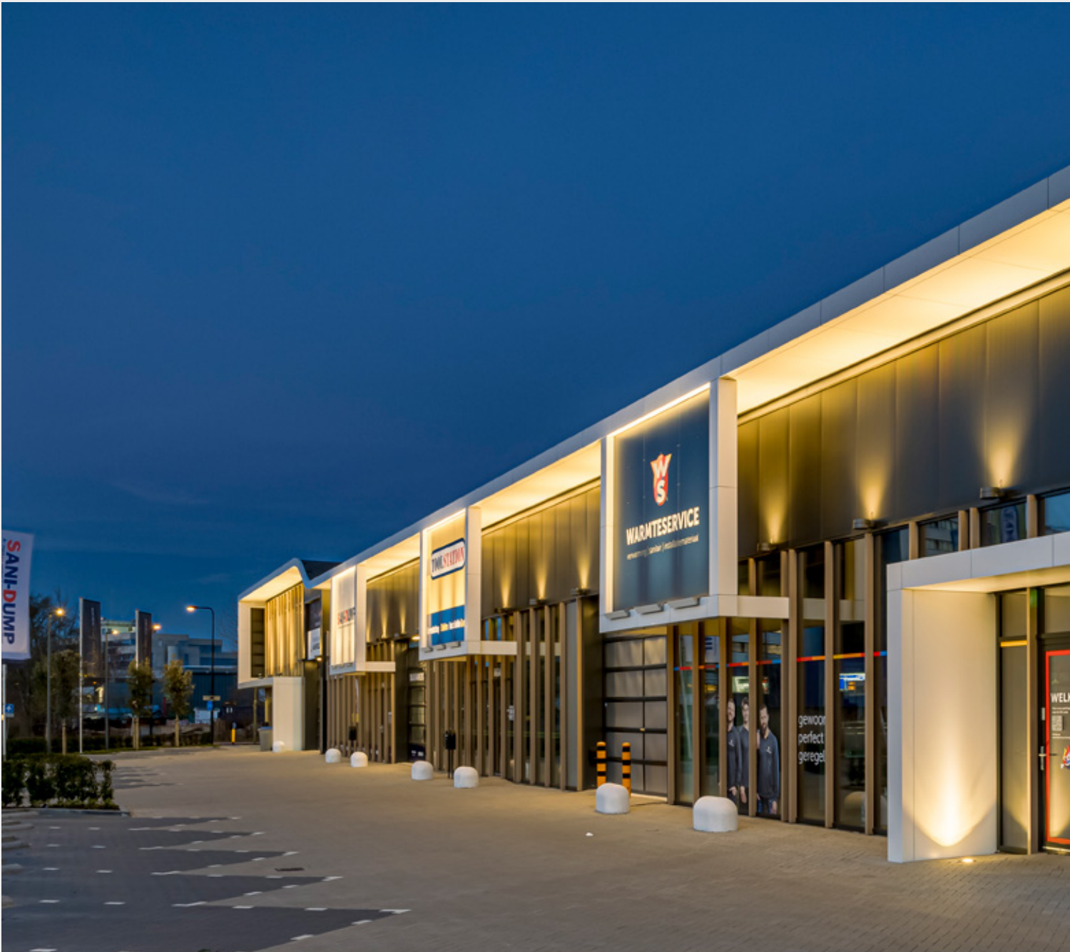
Commercial building Warnteservice | Gouda | Netherlands
