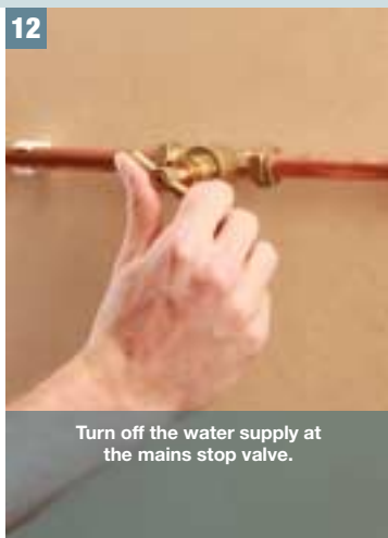
Note: We recommended that a WRAS listed isolating valve be fitted between the rising main and the unit for any future service needs without having to turn off the house water at the stop valve.
