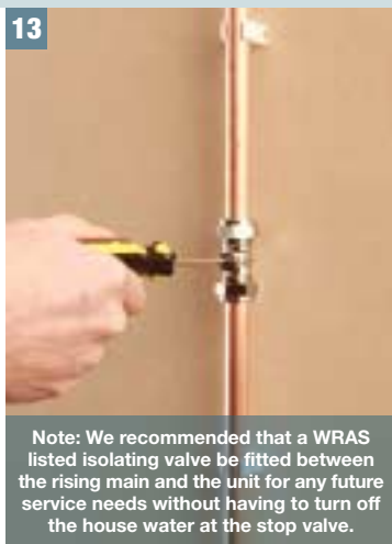
Connect the mains water supply to the Inlet of the shower via 15mm copper, stainless steel or plastic pipe using a 15mm compression fitting. Plumbing - Bottom Entry Option.
