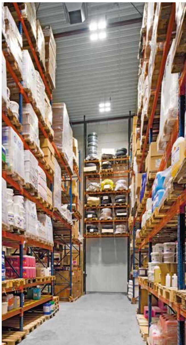
Sigron Warehouse, Vienna, Austria
