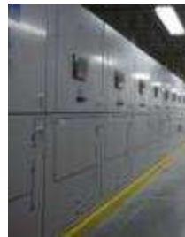
Paralleling switchgear
