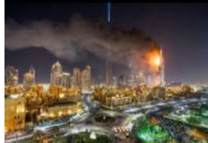
Hotel 63-Storey a Dubai in fiamme
