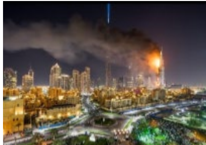
Hotel 63-Storey a Dubai in fiamme
