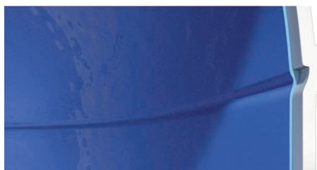
Internal coating of the tank with CRYSTAL PROTECT tech
