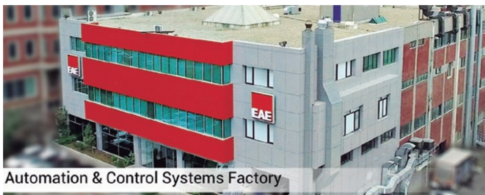
Figura 4. Automation & Control Systems Factory. 25 000 m 2 Istanbul - Turquia.
