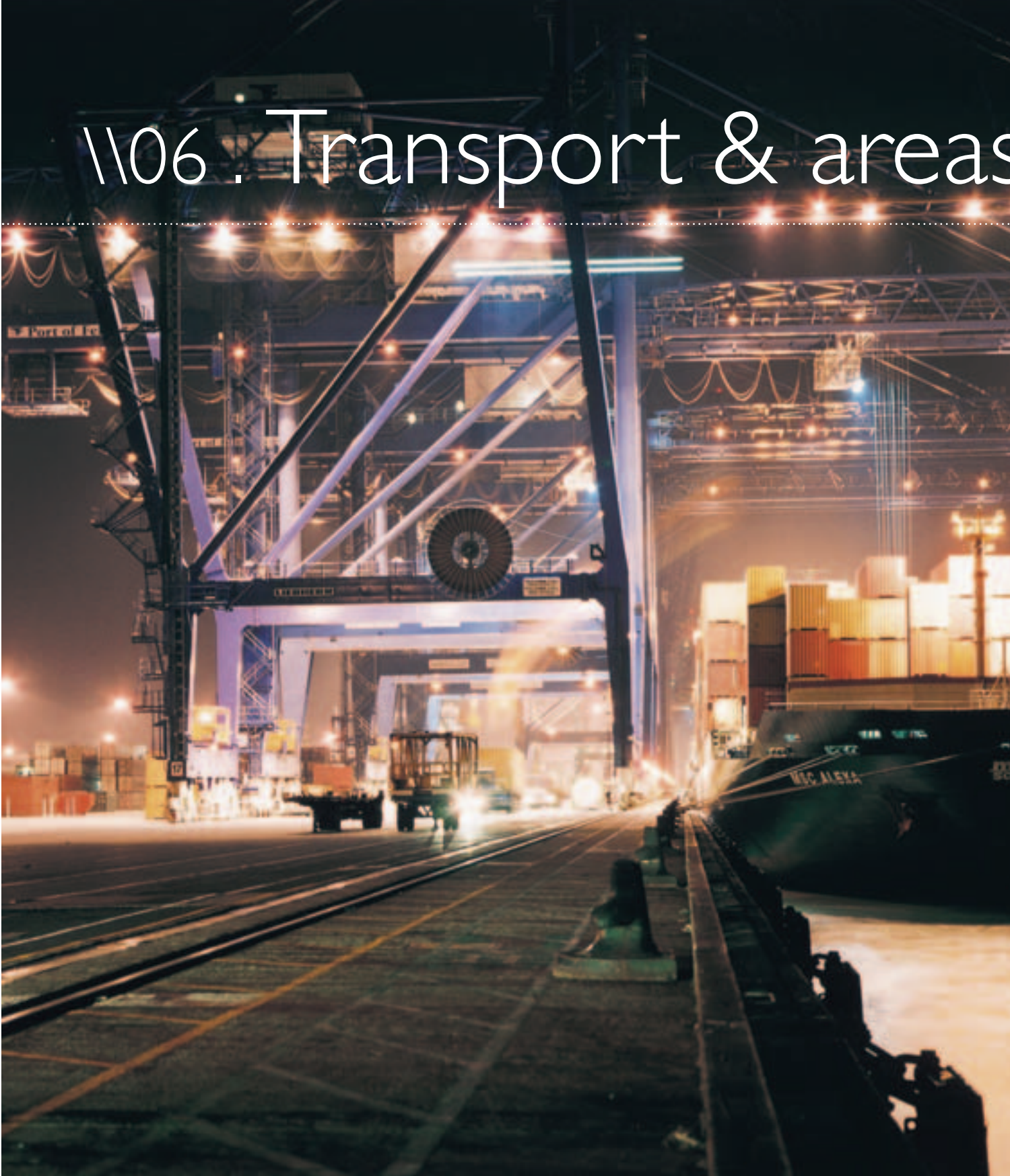
Container Terminal, Felixstowe, United Kingdom
