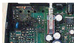
Example: Damage on a modem motherboard due to atmospheric surge carried by the telecom line.
