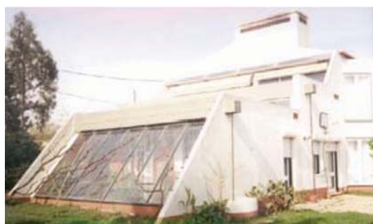
Figure 3. “Vale Rosal Building (Charneca da Caparica-Lisbon). Gonçalves et al. 1997.
