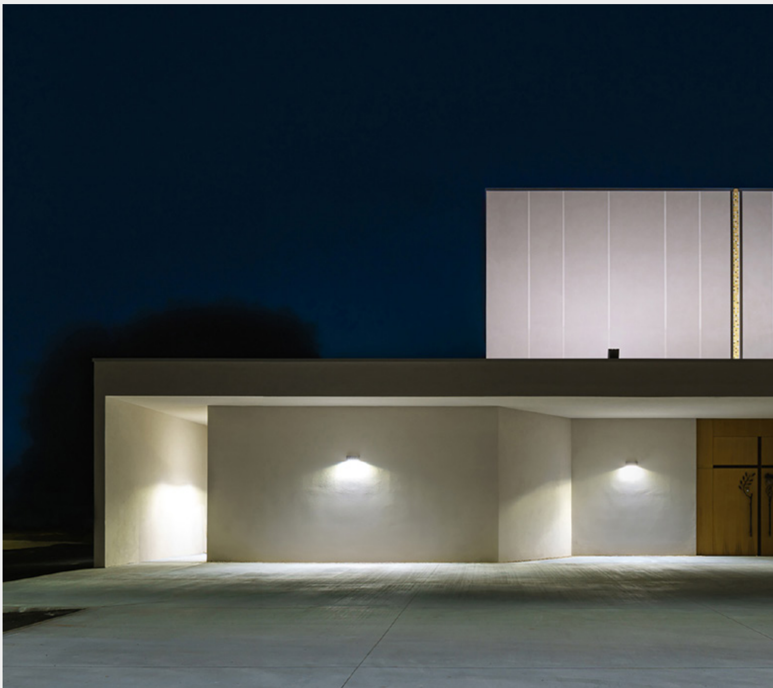
Parish Complex | Varignano - Viareggio | Italy
