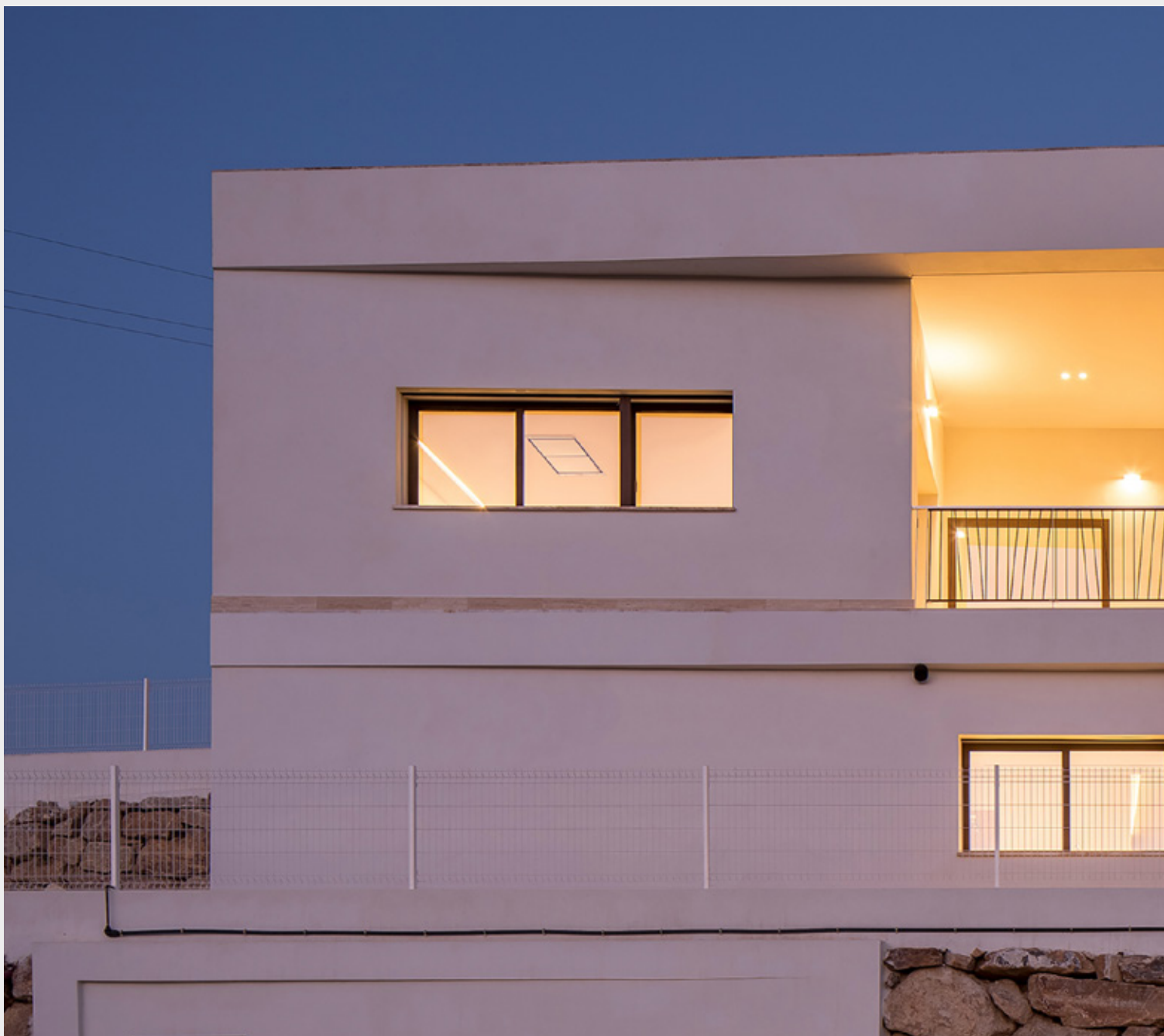
House in Albánchez | Almería | Spain
