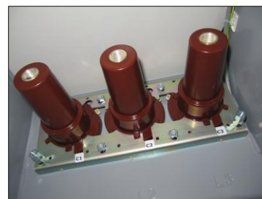
Cones type C Load-break switch 630 A without current transformers
