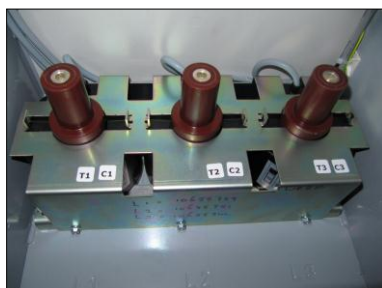
Cones type A Circuit-breaker 200 A incl. current transformers
