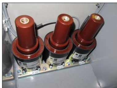
Cones type C Circuit-breaker 500 A incl. current transformers
