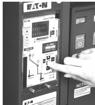
VCP-T/VCP-TL Circuit Breaker with Integral Protective Relay
