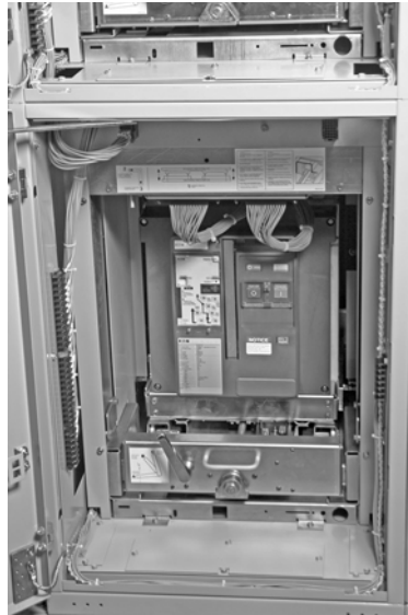
Circuit Breaker Compartment— Breaker in Connected Position
