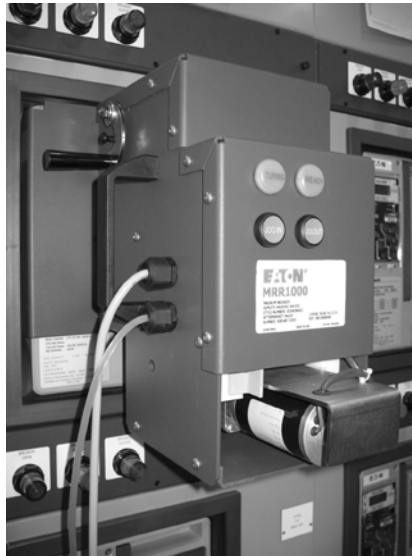
MRR1000 Connected to Magnum Breaker
