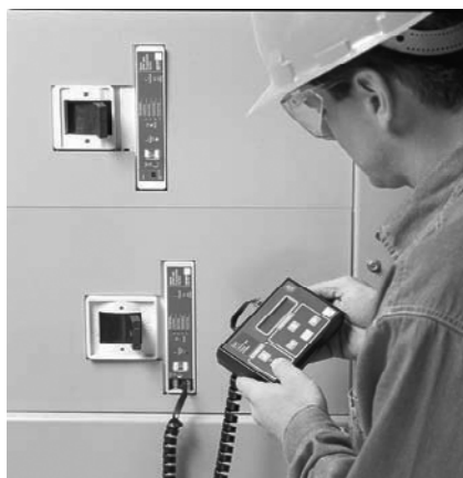
Commissioning of Electrical Services
