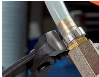
10 98 I220: Sealing the hose connection on central lubrication
