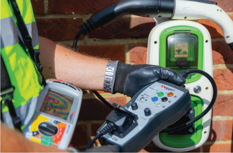
Testing a New Charge Point Installation
