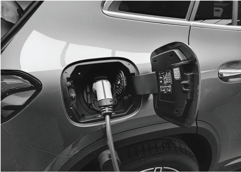
Electric Vehicle Connected to a Charge Point
