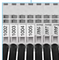
Clear terminal block identification Top large marker. Hand pre-marking before final marker installation
