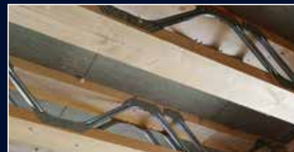
Metal Web Joists
