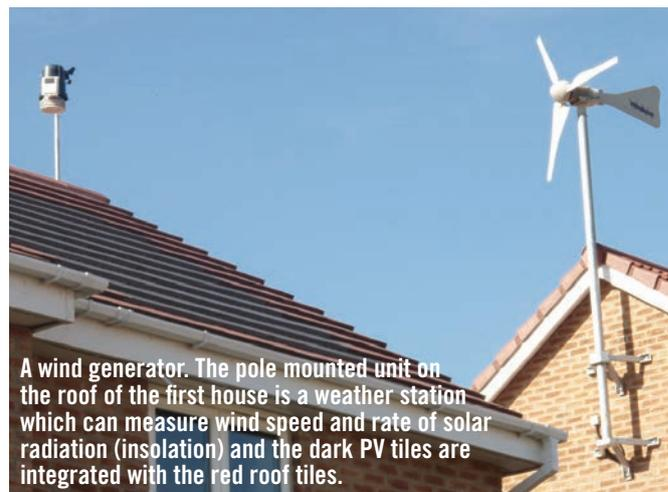
A wind generator. The pole mounted unit on the roof of the first house is a weather station which can measure wind speed and rate of solar radiation (insolation) and the dark PV tiles are integrated with the red roof tiles.
