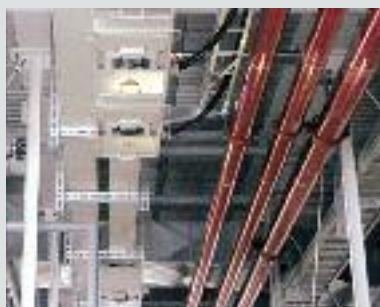
Busbar trunking saves space in riser shafts and allows simple later expansion by plugging in a new tap off unit.
