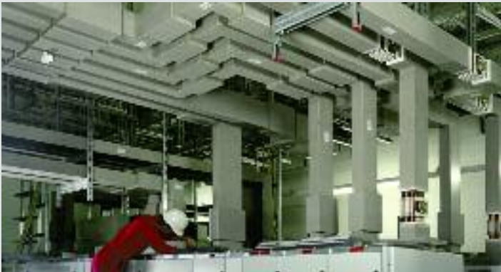
Compact size, high IP rating busbar can carry large current ratings through the most difficult environments.
