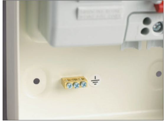
16mm Earth terminating point inside enclosure
