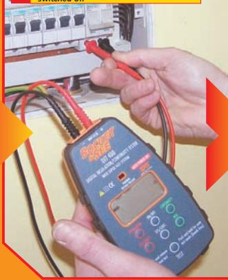
Repeat this test with connections to the two neutral conductors (black or blue) (Fig. 6), with results that should be about the same as for the phase ring. A further test on the earth ring should result in values about 66% greater than those for the phase and neutral because the earth conductors have smaller cross-sections.
