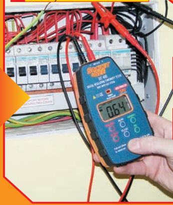
Next, go to each socket outlet, remove it from its box (Fig. 7) and test the resistance from phase to neutral on each (Fig. 8).
