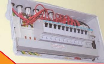
Turn off the main isolator at the consumer unit. Check that the system has really been switched off. With the tester SWITCHED ON carefully put the probes on the terminals at the live side of the mains isolator.
